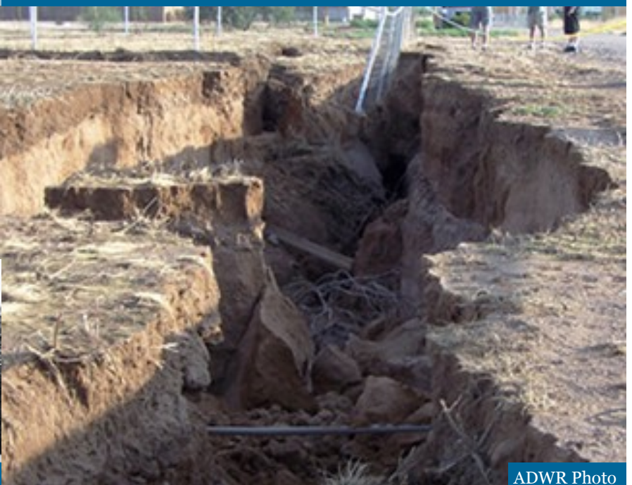
Earth fissuring due to groundwater over pumping in an area prone to subsidence
