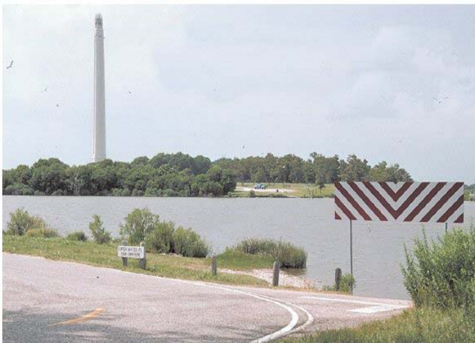
A road that provided access to the San Jacinto Monument was closed due to flooding caused by subsidence.
